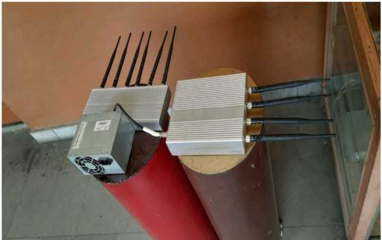
Jammer installed during examination
